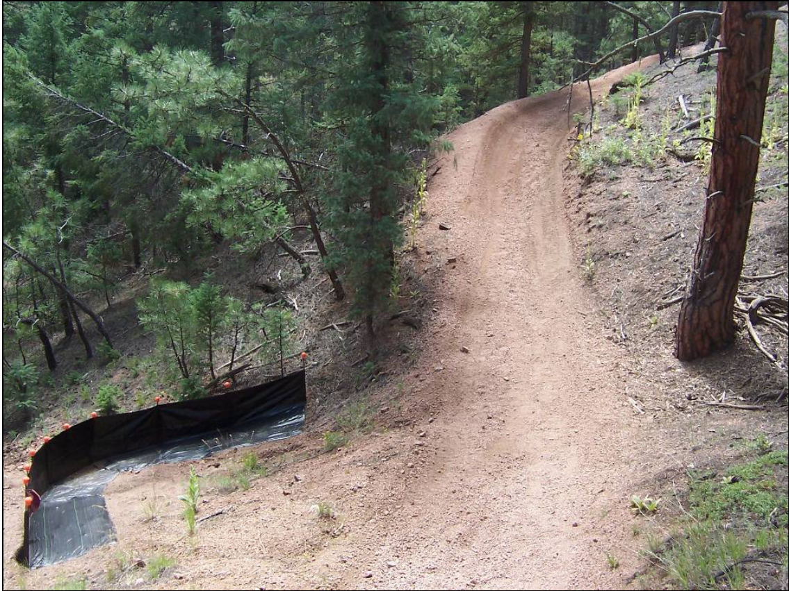
Figure 3.2. A sediment fence installed below an OHV trail segment at the Log Jumper study site. Note the incision into the hillslope at the upper end of this segment.
