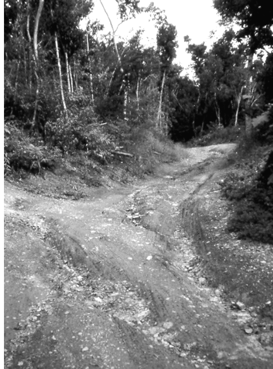
Figure 2. Example of a steep road segment near Bordeaux Mountain with a deeply-rilled travelway.
