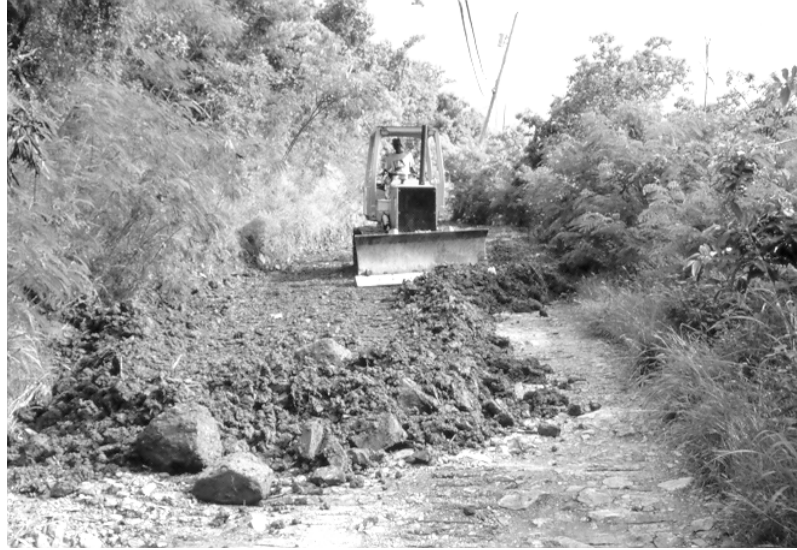
Figure 8. Example of a grading operation along road segment FB-Coco on 11 December 1998.
