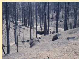
Figure 1. Sediment fence in the axis of a swale.
