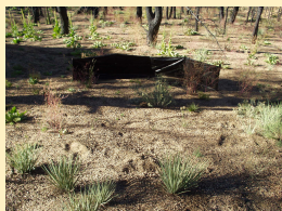
Figure 1. Sediment fence on a planar hillslope.
