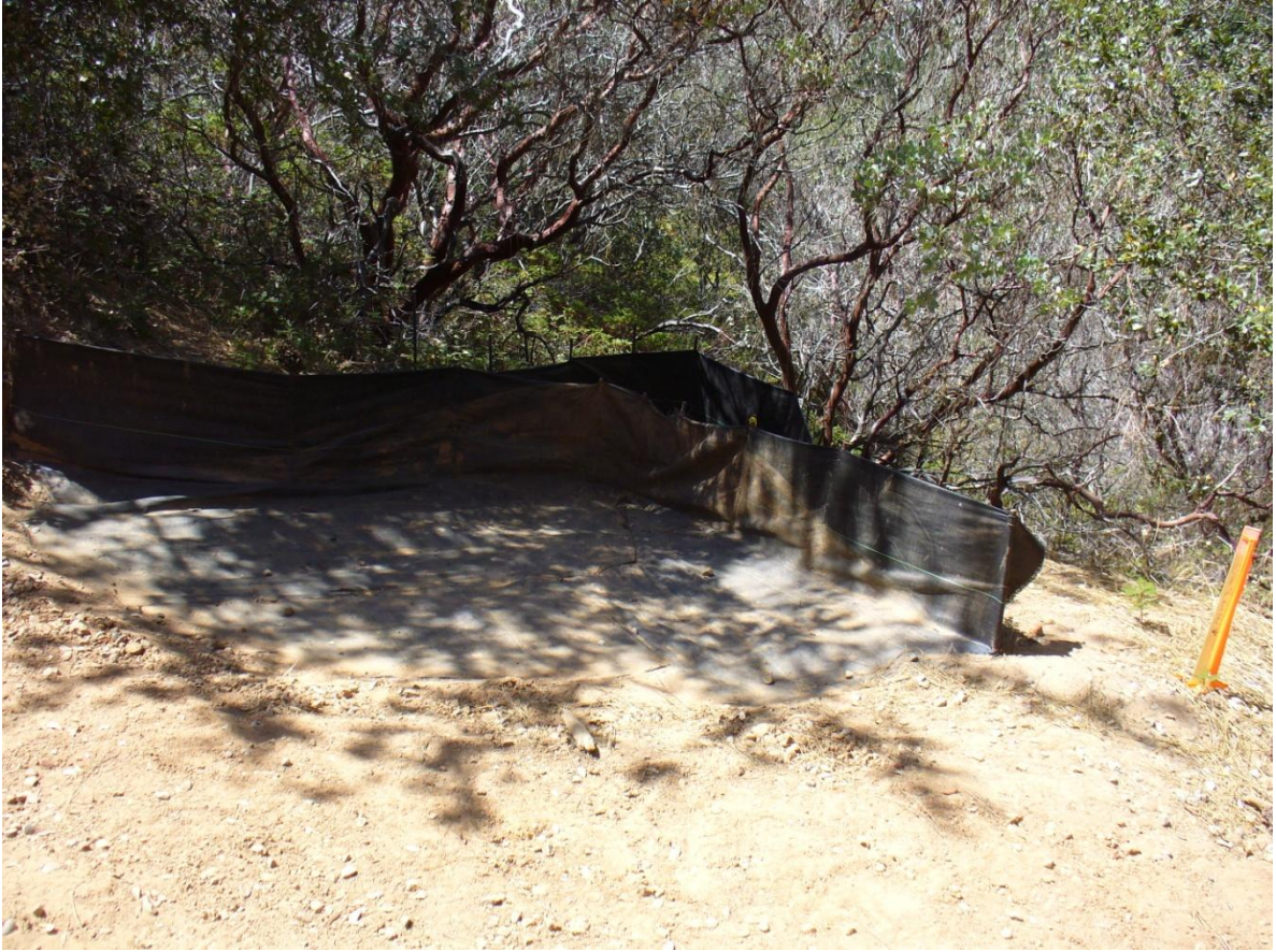
Figure 3.4. One or more sediment fences were installed at the drainage point of road segments in José Basin and the Providence Creek watersheds. The fence in the foreground was installed in summer 2007 in José Basin just below a waterbar draining a native surface road segment, and the second fence was added in summer 2008 to prevent overtopping.
