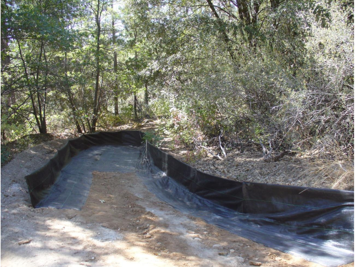
Figure 2.6. Sediment fences were installed at the drainage point of native surface road segments in José Basin as well as the Providence Creek and Bull Creek watersheds. This fence was installed just below a waterbar draining a native surface road segment in José Basin in summer 2007.
